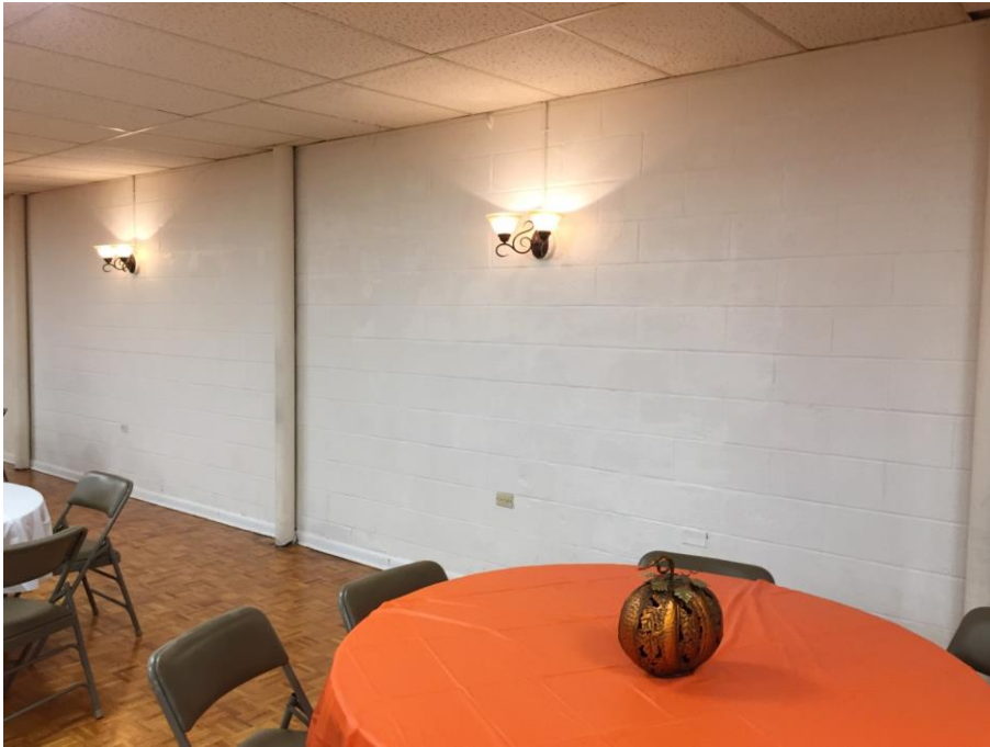
The wall after first coat of new water proof paint
