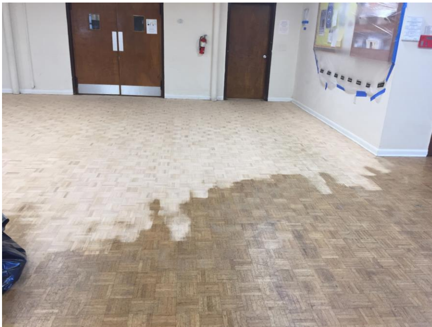
Wooden floor in the process of being renovated.
